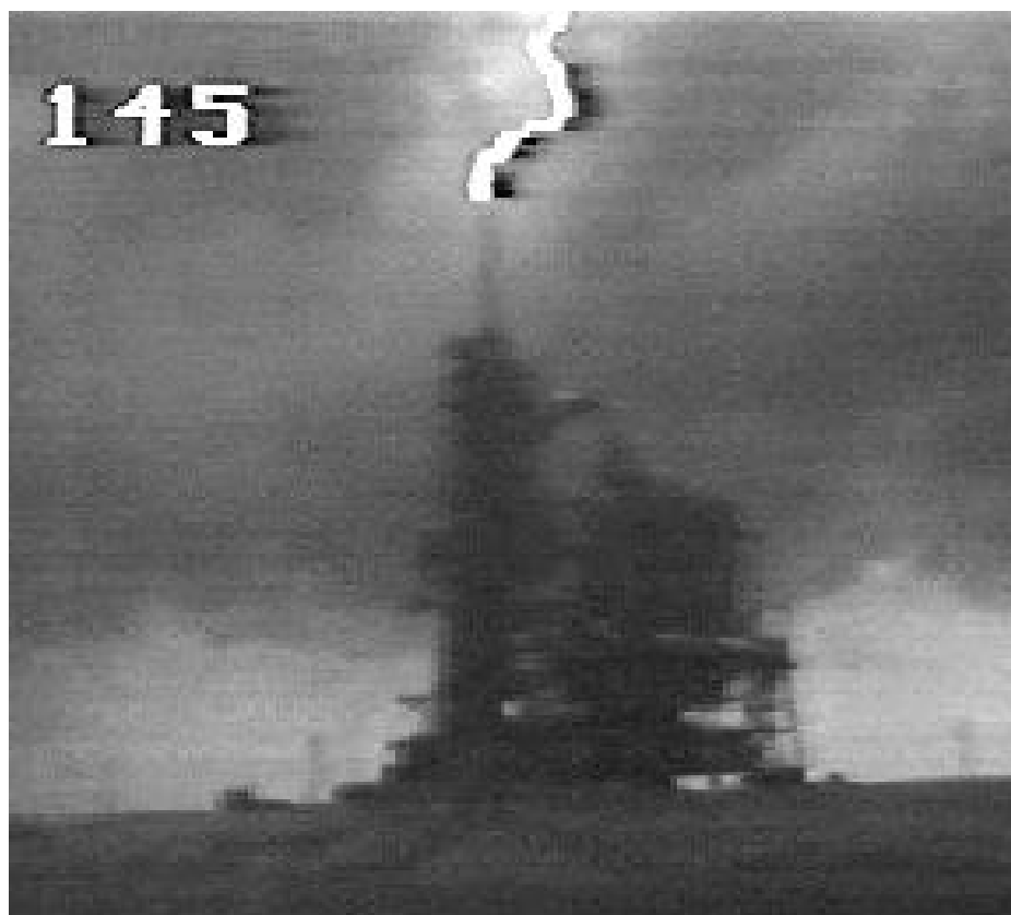
Figure 10. Lightning Strike to Launch Complex 39, Kennedy Space Center, Florida. The air terminal protecting the shuttle on the pad intercepted the strike.
