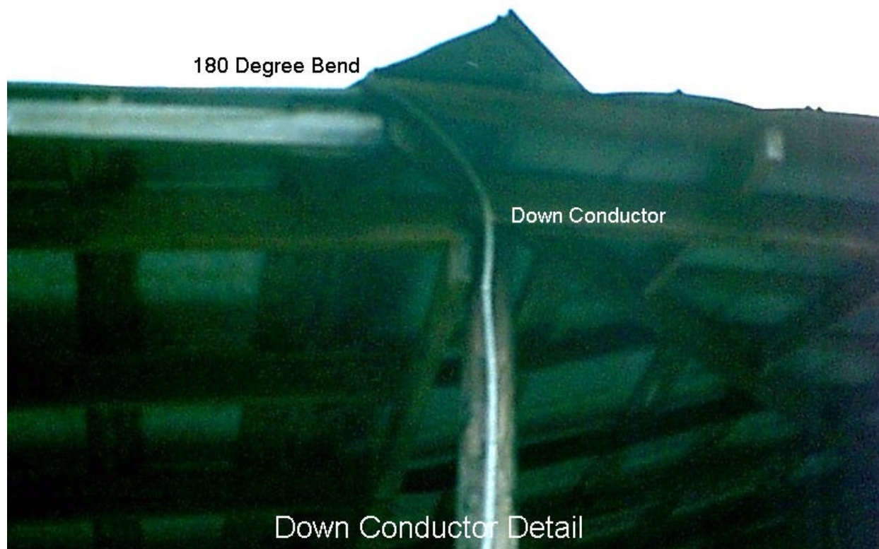
Figure 7. Detail of 180 degree bend on farm shop.
